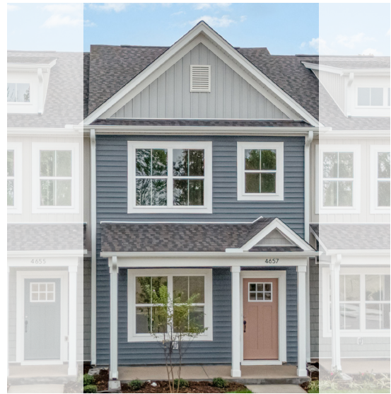
THE IRVINE II INTERIOR UNIT
